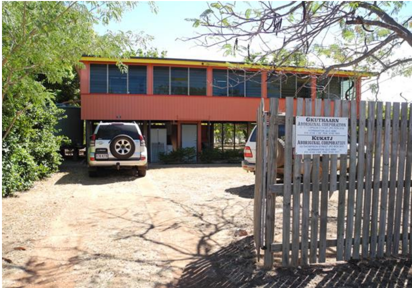
Figure 4: Gkuthaarn and Kukatj building in Normanton rented by Century as a CLO office at the time of the community consultations in 2012.
