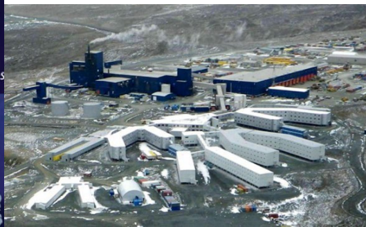
Image 16 – Raglan mine infrastructure
